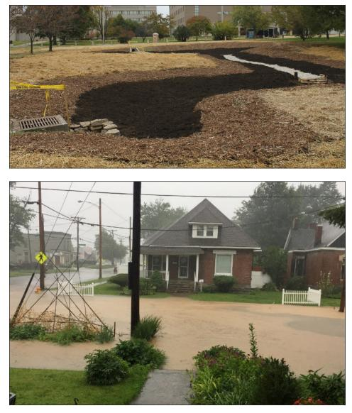
**Figure 10.** Installing erosion control measures, such as straw and mulch, is a critical yet often overlooked aspect of constructing an outdoor classroom (top). If left unprotected, rainfall will easily erode bare soil, which is then transported offsite in the form of runoff (bottom).
