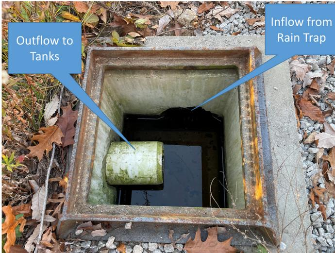
**Figure 6.** A catch basin collects the flow in one location, provides a chance for sedimentation to occur, and transfers the collected water to storage. The catch basin also includes a trash grate, which was removed for the photo.
