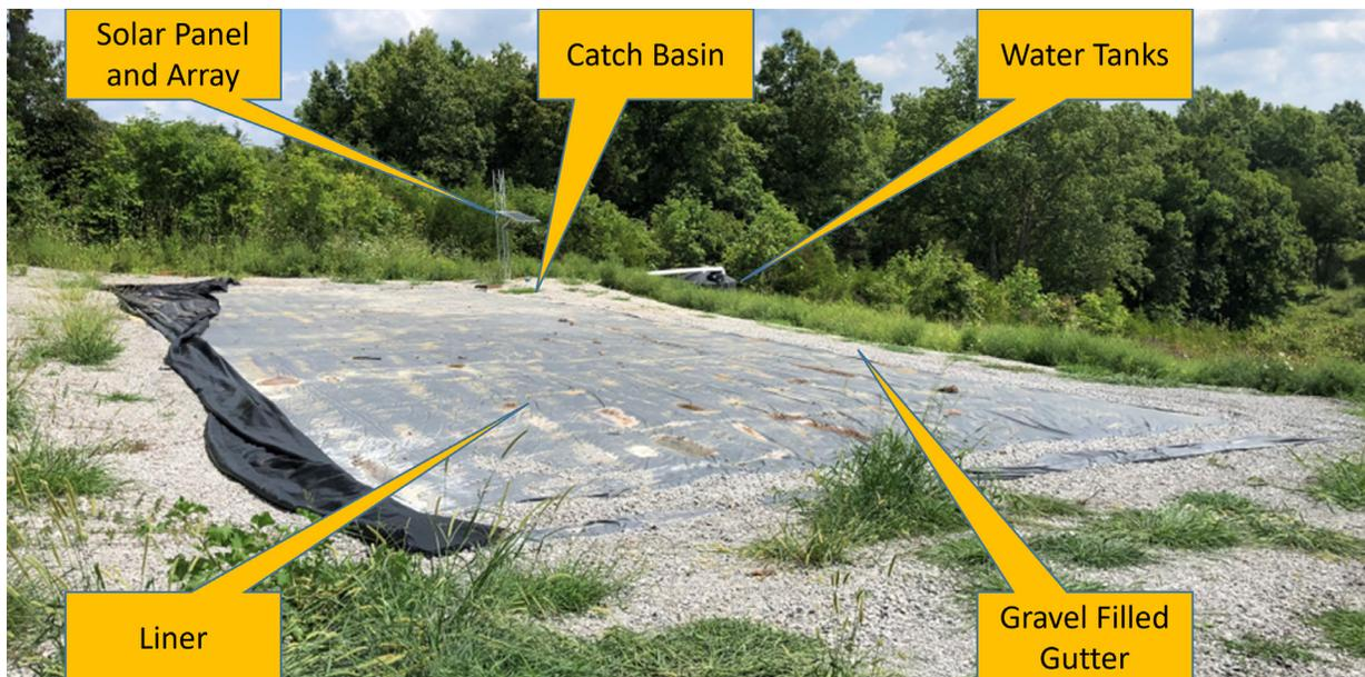
**Figure 5.** The rain trap area after construction, during which the brush and trees were removed and the land was graded to create the final surface for the trap. In the background is the solar panel and array used to power the water pump system. The top of the water tank, which stores a portion of the collected water, can barely be seen. A second water tank was added the following year.
