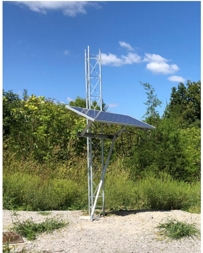
**Figure 7.** A solar-powered pumping system is a useful tool for remote locations. This one is used to pump collected water to a livestock waterer located 275 feet away and 40 feet higher in elevation. The iron grate in the foreground covers the catch basin.
